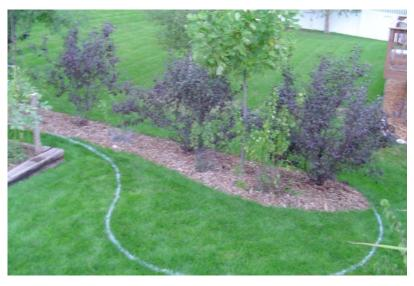
paint or flags. Remember, the size was determined using an average 1 inch storm so if you need to make it slightly bigger or smaller, that's fine. It will either hold a little more or a little less runoff. The garden will have an inflow area where runoff will enter and an outflow area in case you receive more rain than the garden is designed for. Identify these 2 spots when laying out your rain garden. This is where you will incorporate some rocks.
