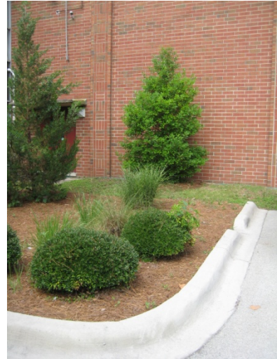
Downspout disconnection to pervious pavement and bioretention area
