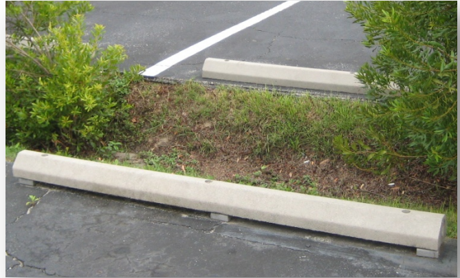
Figure 4. Parking stops were raised post retrofit to avoid flooding (WECO).
