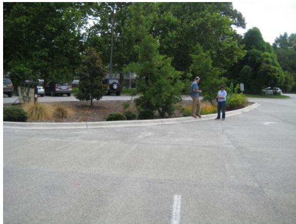
Pervious pavement and bioretention area
