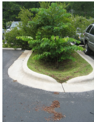
Allowing parking lot water to flow into bioretention area
