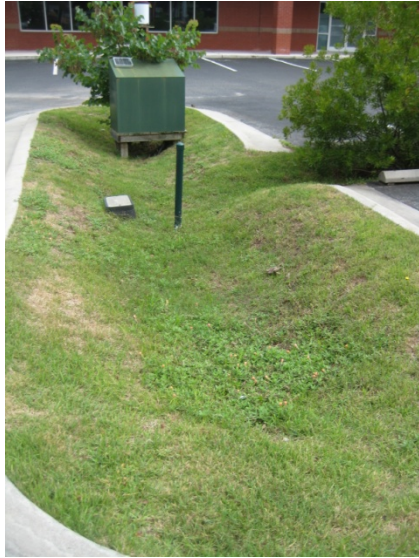
Bioretention area before a sampling point
