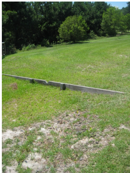
Weir slows down stormwater runoff sheetflow
