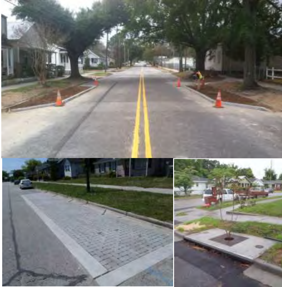
Figure 2-2: Clockwise from top: BRC bumpouts along Dock Street, tree filter device at intersection of 12 th Street and Dock Street, and permeable pavement parking stalls on 12 th Street
