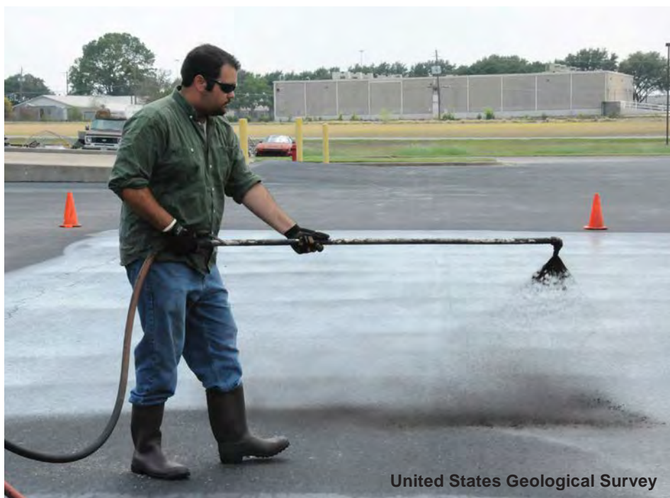
Figure 3. Sealant is applied to a parking lot.
