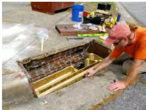
Figure 13: V-notch weir and weir box being installed inside existing catch basins for the street retrofit project
