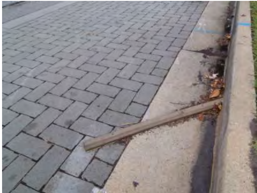
Figure 2-3: Flow diverters installed on permeable pavement parking stalls along curb and gutter of 12 th Street
