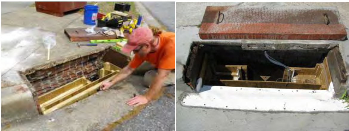
Figure 2-6: V-notch weir and weir box being installed inside existing catch basins
