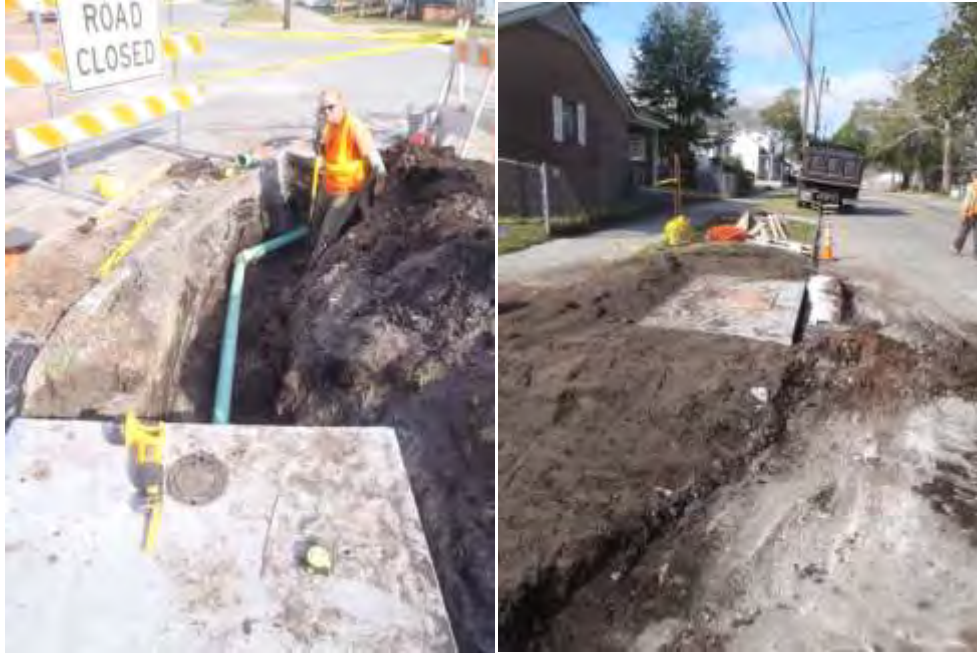
Figure A-5: Filterra® unit underdrain installation
