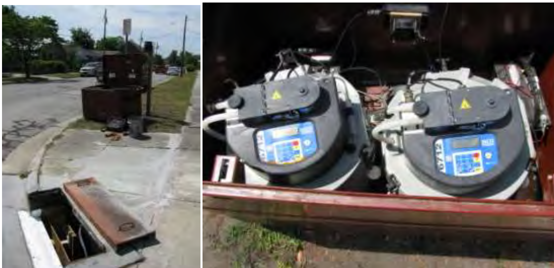
Figure 3-7: Retrofit station with JoBox™, rain gauges, and weir box inside existing catch basin (left), two ISCO 6712™ portable samplers with ISCO CDMA Cellular Phone Modem™ installed inside retrofit JoBox™(right)
