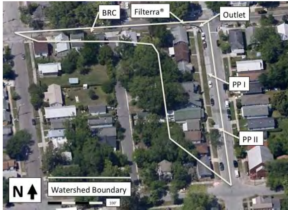
Figure 7: Aerial photo post-retrofit with approximate drainage area boundary
