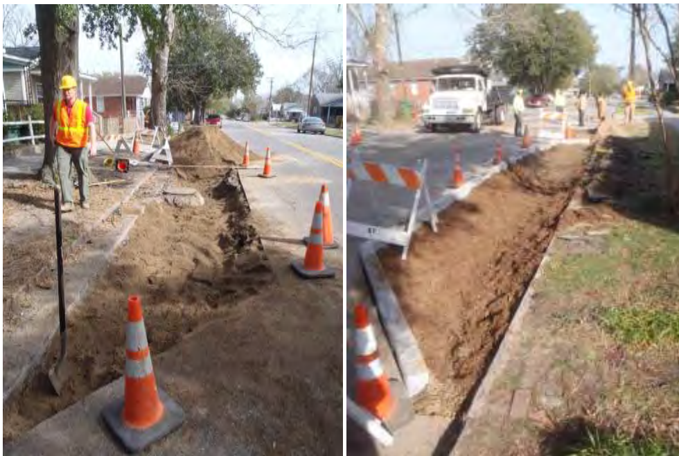
Figure A-2: BRC media and mulch installation on Dock Street
