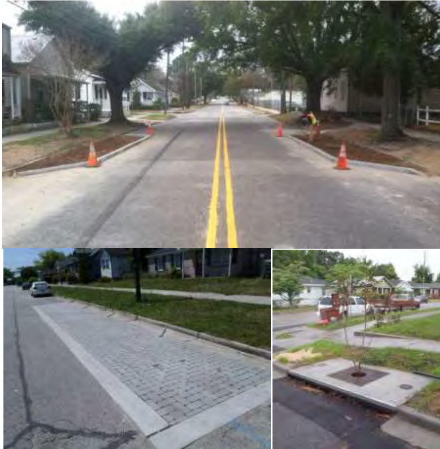
Figure 3-2: Clockwise from top: BRC bumpouts along Dock Street, tree filter device at intersection of 12 th Street and Dock Street, and permeable pavement parking stalls on 12 th Street
