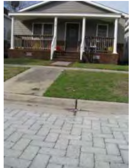
Figure 3: Permeable parking on 12th St.
