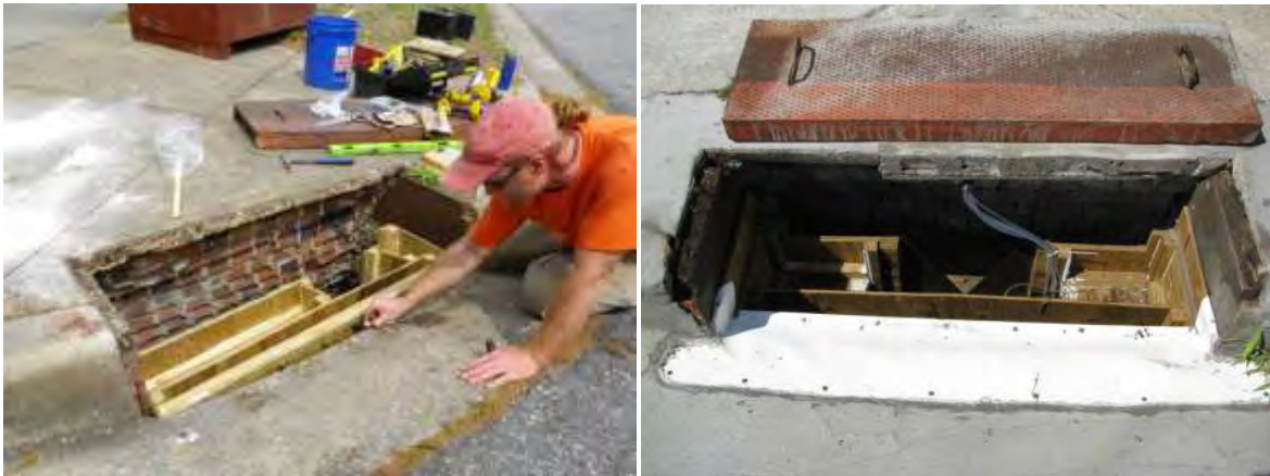
Figure 3-6: V-notch weir and weir box installed inside existing catch basin
