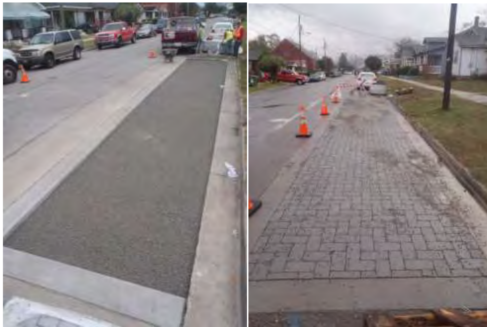
Figure A-8: #78 stone placement and recently installed PICP pavers
