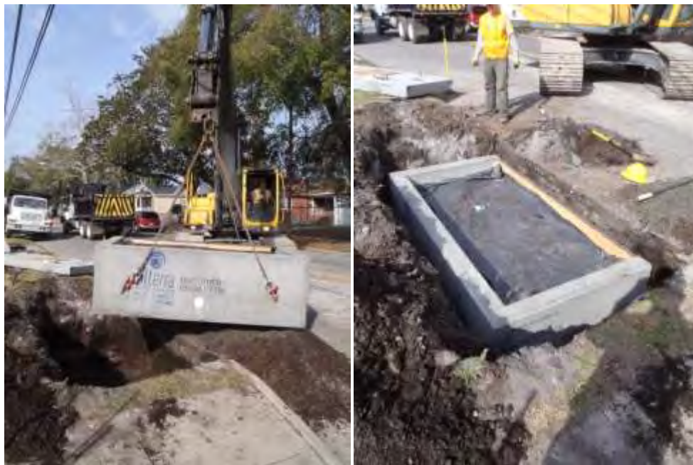
Figure A-4: Filterra® unit installation at the intersection of 12 th Street and Dock Street
