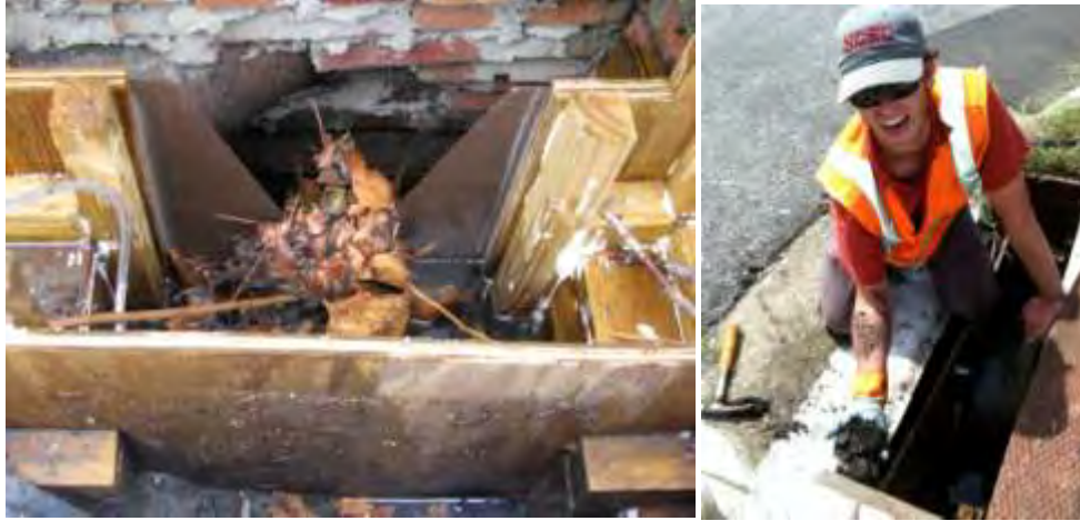
Figure 3-9: Debris clogging control weir (left) and removing organic material from control weir box (right)
