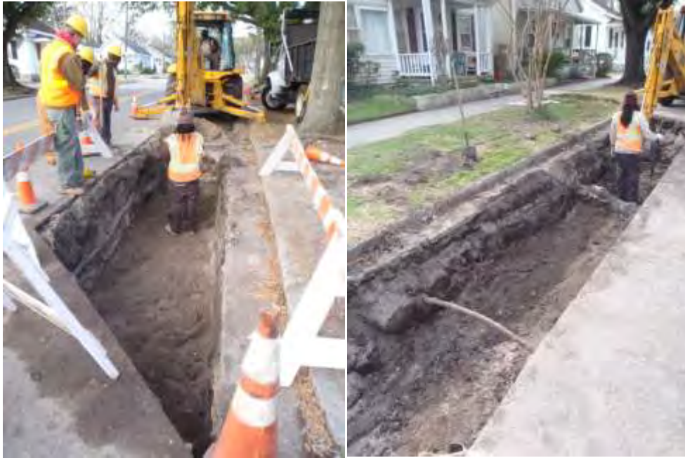
Figure A-1: BRC excavation on Dock Street and existing utilities
