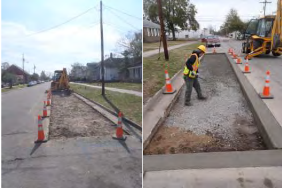
Figure A-7: Permeable pavement excavation and #57 stone placement
