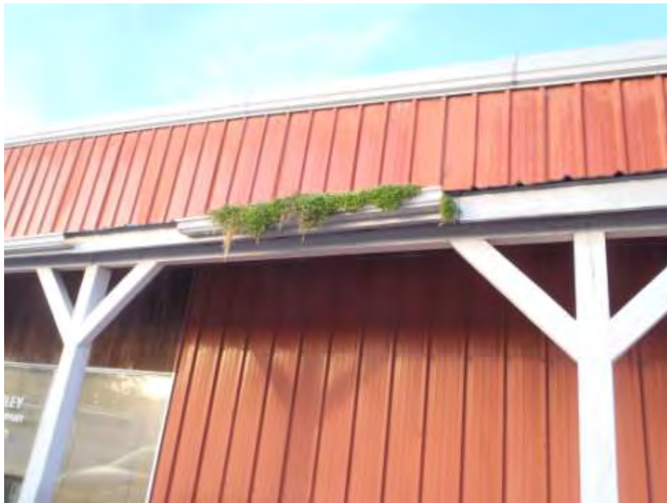
Figure A-10: Coastal North Carolina green roof
