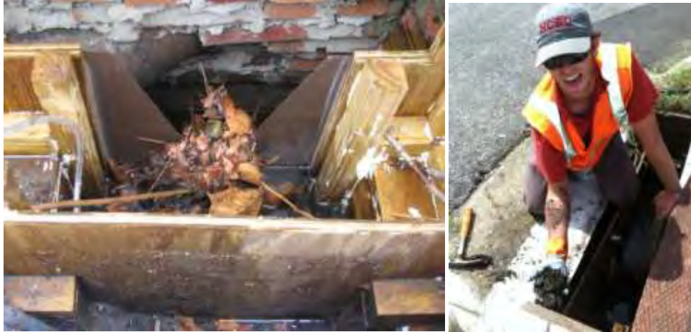
Figure 2-7: Debris clogging control weir (left) and removing organic material from control weir box (right)
