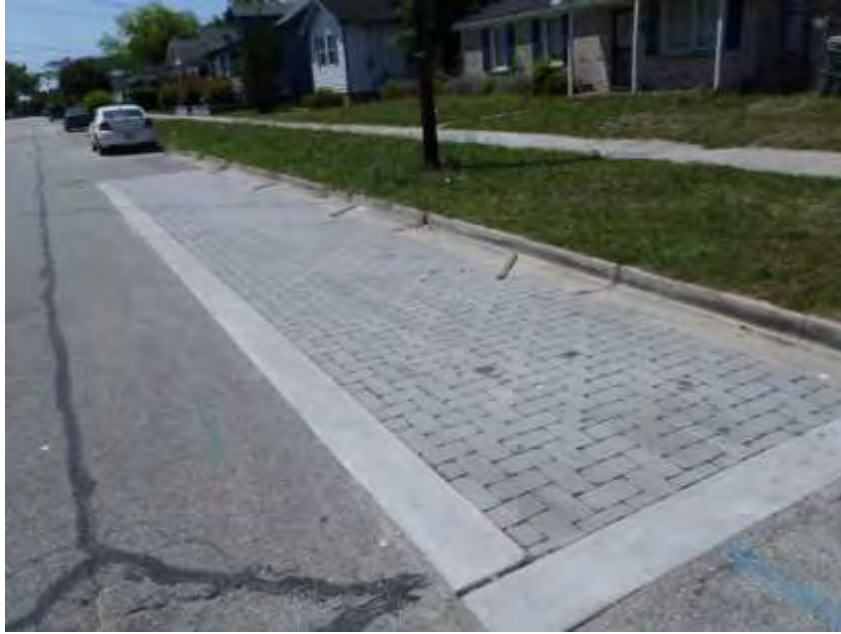
Figure A-9: Completed permeable pavement parking stalls with flow diverters along existing curb and gutter
