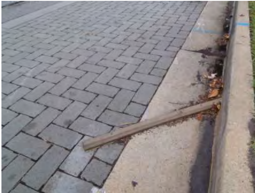
Figure 3-3: Flow diverters installed on permeable pavement parking stalls along curb and gutter of 12 th Street
