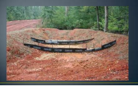
2. INSTALL ADEQUATE SEDIMENT STORAGE DEVICES
