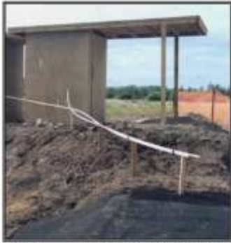
Figure 4. Rainfall Activated Flocculation Housing
