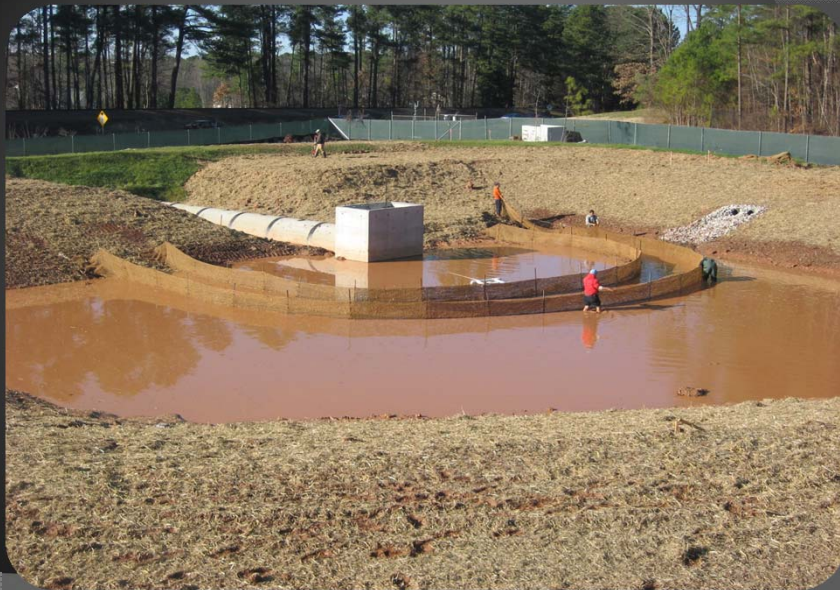
SITE CHALLENGES Erosion Control Measures
