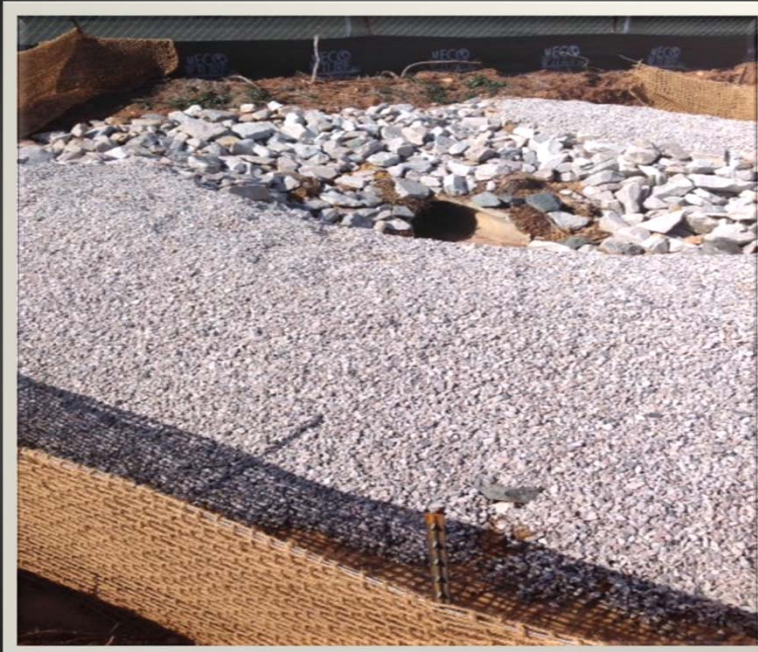
Rock Inlet Protection
