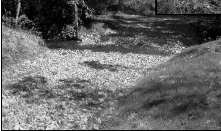
Ford crossing, ample ballast on each approachway and side banks grassed-over, Franklin Co.
