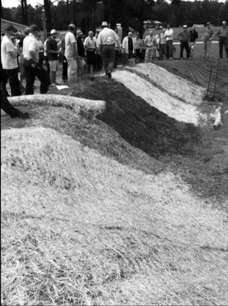
Erosion Control Matting slopes & stream banks
