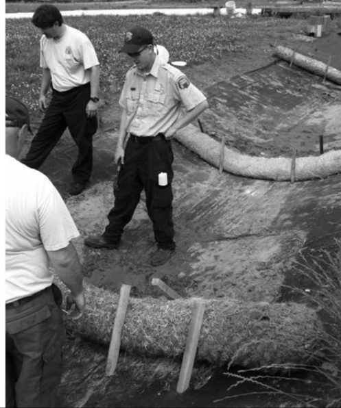
Coir / Fiber Logs, or "Wattles" fiber check-dam, instead of rip-rap
