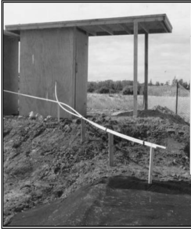
Figure 4. Rainfall Activated Flocculation Housing
