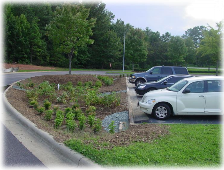
Figure 4 West Cary Middle school parking lot with bioretention
