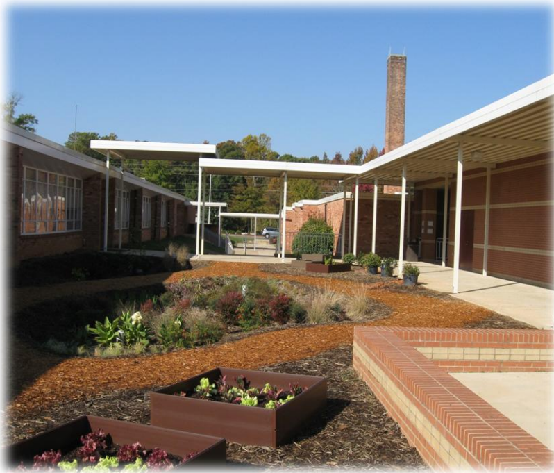
Figure 6 West Cary Middle courtyard with bioretention cells and gardens
