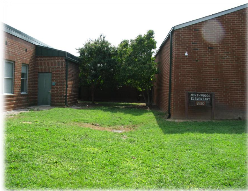
Figure 7 Northwoods Elementary courtyard before
