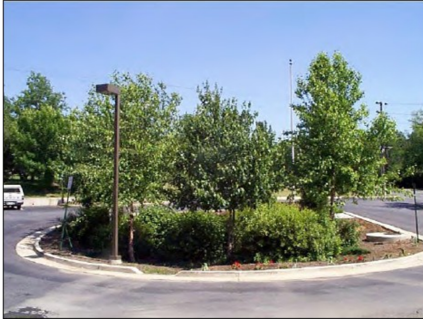
Figure 7: Introduction (Subwatershed Health and Restoration) - Bioretention. Smaller BMPs and LID practices, such as bioretention or rain gardens, can be implemented for a cumulative effect. (Schueler et al 2007)
