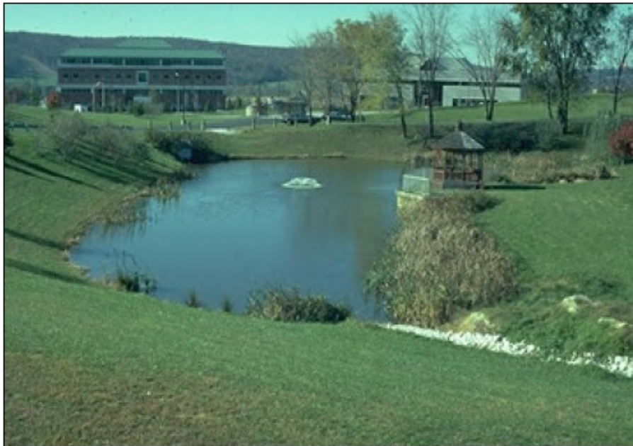
Figure 6: Introduction (Subwatershed Health and Restoration) - Stormwater Wet Pond. Best Management Practices (BMPs) can isolate, retain, and handle larger subsets of stormwater runoff. (Schueler et al 2007)
