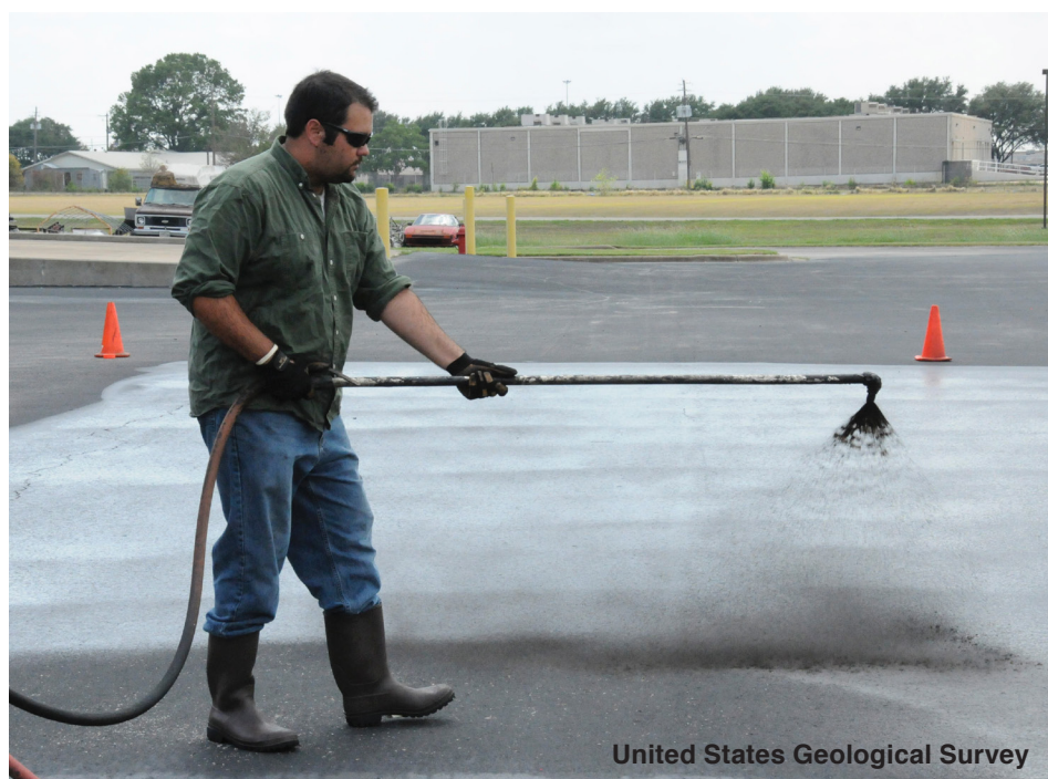
Figure 3. Sealant is applied to a parking lot.
