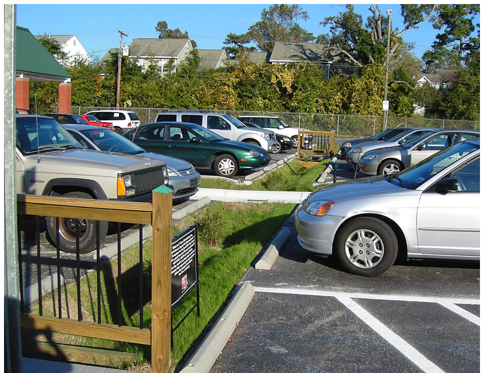
Figure 5. This bioretention cell reduced PAHs in runoff flowing through it.
