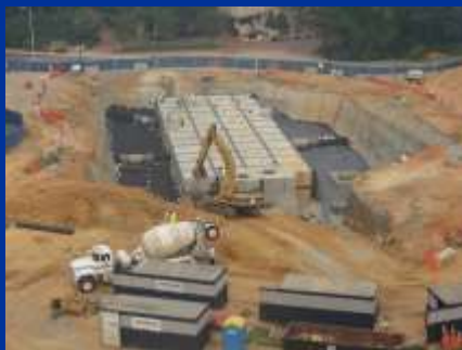
Cistern Start and Sealing
