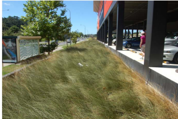
Rooftop Treatment in Albany, NZ (Courtesy Bill Hunt)
