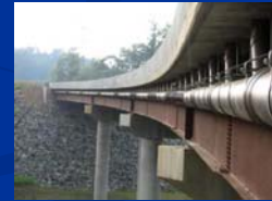
Stormwater collection system on U.S. 64 bridge over the Hiwassee River in Cherokee County, North Carolina
