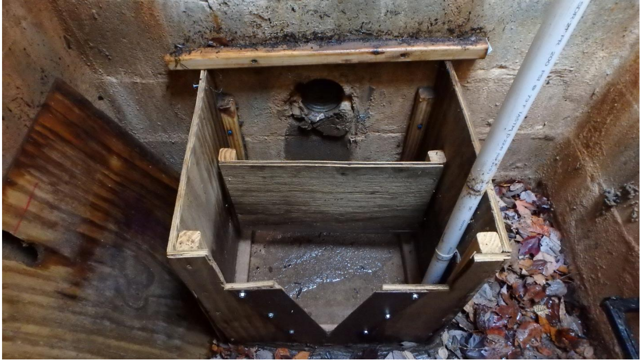
Figure 5. Pre-retrofit underdrain entrance to DT outlet structure.
