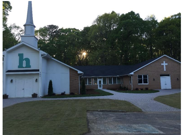
Figure 6: Harvest Church permeable walkways and bioretention
