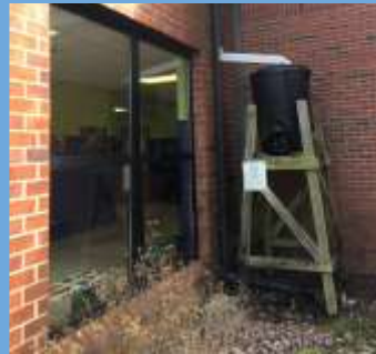
Rainwater Recovery Cistern
